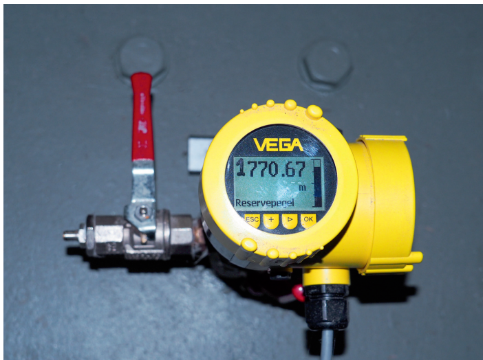
VEGABAR 82 takes on the task of redundant measurement, determining the water level in the reservoir with centimetre accuracy.
